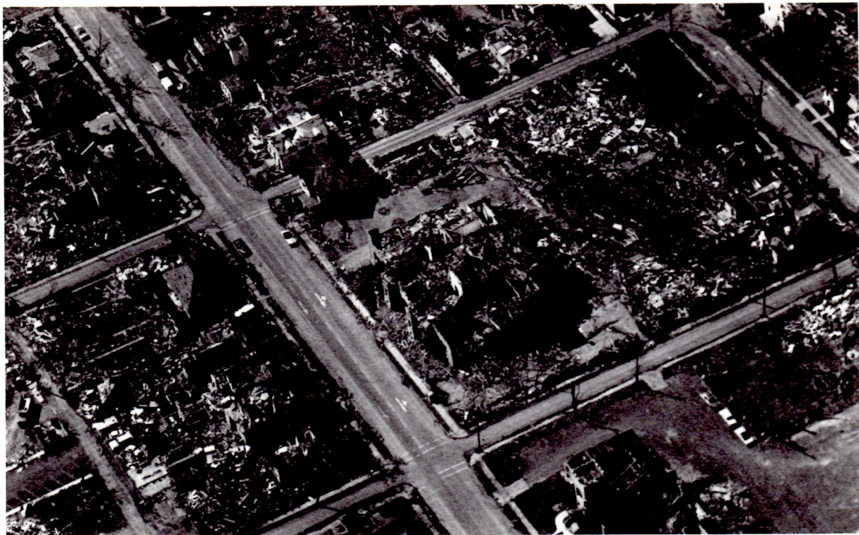
Damage to school and nearby residences.
