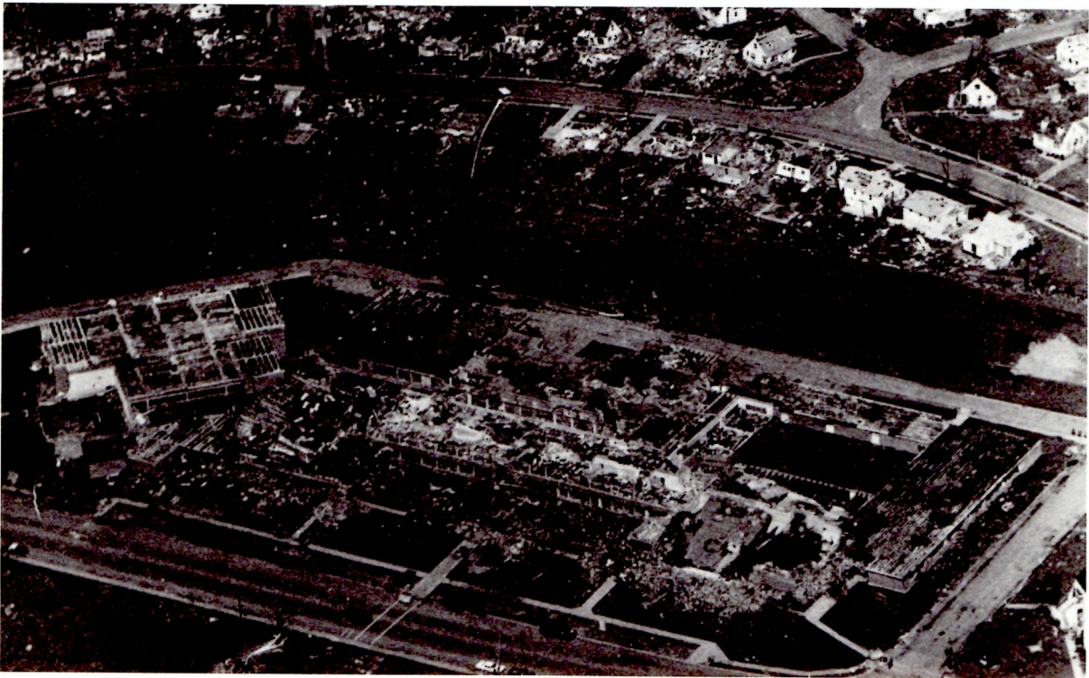
Damage to school and nearby residences.
